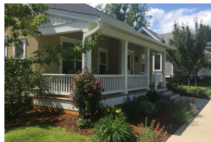
When the porch is located close to the sidewalk, a cluster of layered large and small shrubs and perennials arranged in front of the porch creates an appealing composition. A view from Washington Village in Boulder, Colorado (top); a view from a home in the 12th Street Historic District in Golden, Colorado (bottom).
